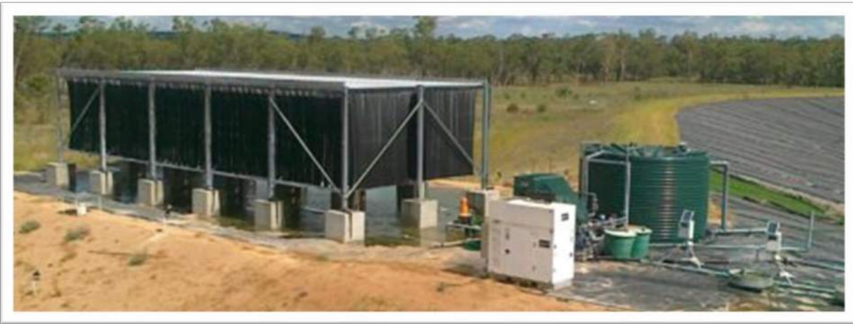
Figure 12 – WAIV Unit Installation
