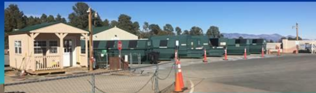
Solid Waste Handling Facility
