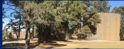
Storage Tank and Booster Pumps
